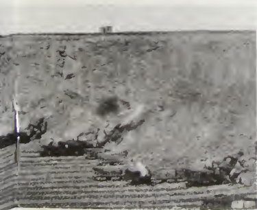
pick up several tons of the blasted rock at each bite.
